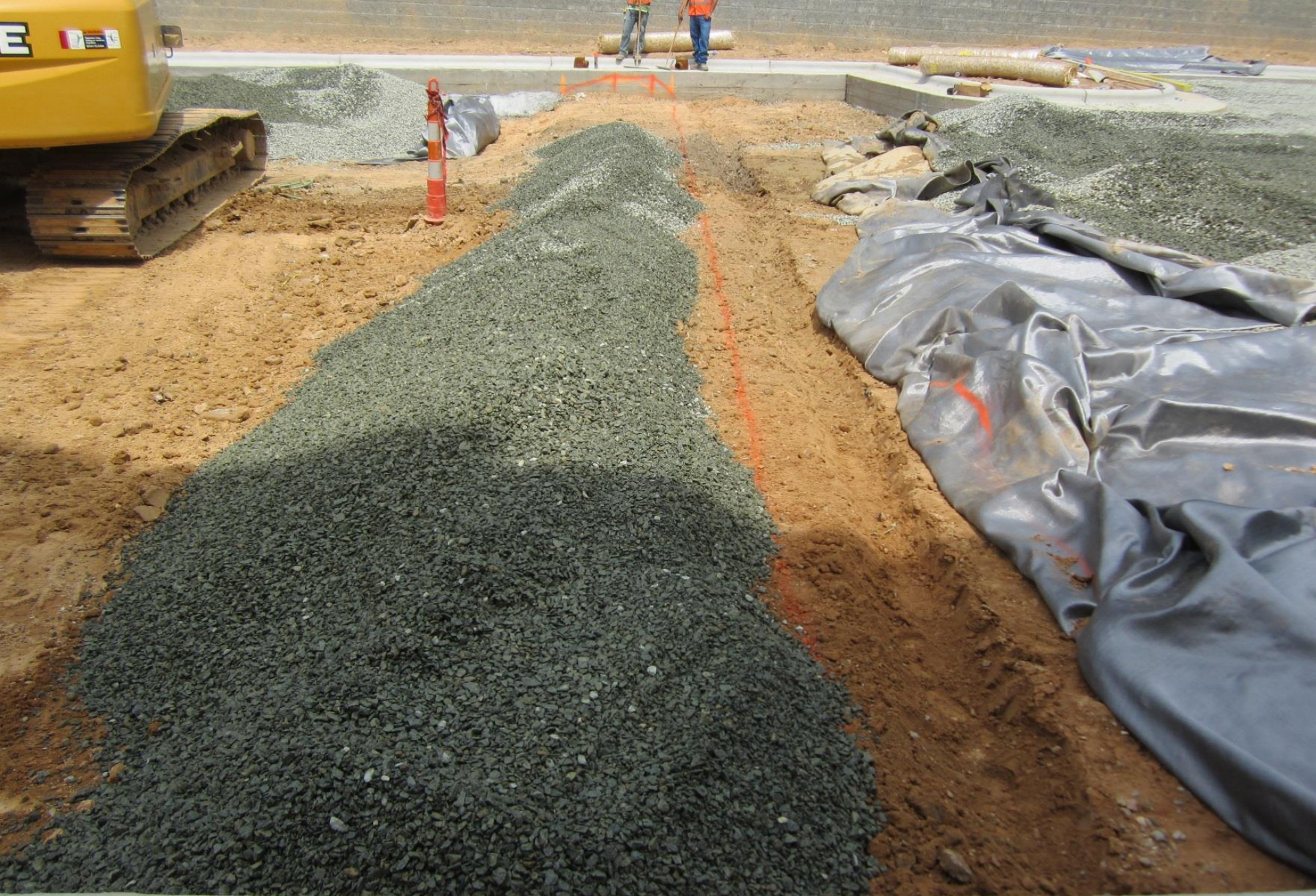
General Baffle Construction
