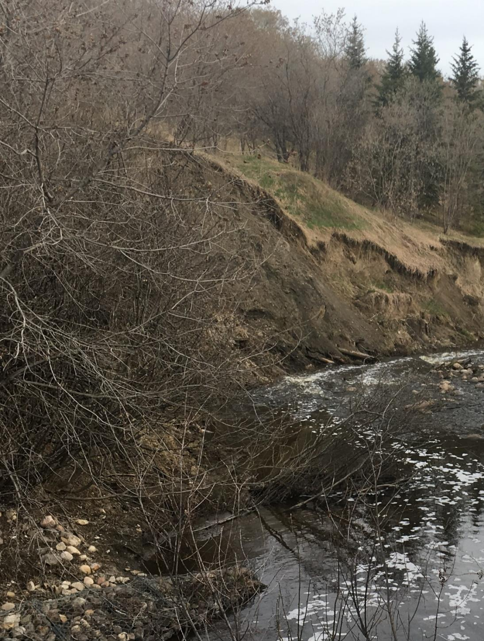
Gabions and Bank Erosion
