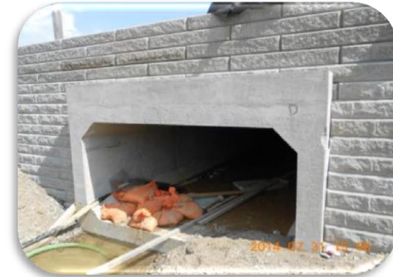
Culvert upgrade – City of Brantford
