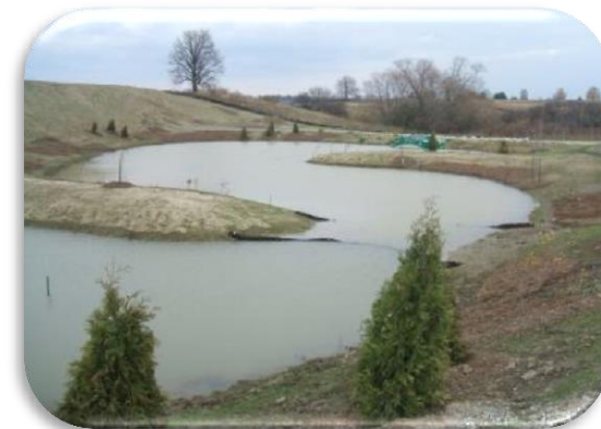
Traditional Stormwater Management Pond
