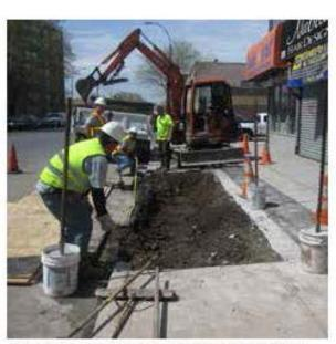
The sidewalk and curb are removed and the material underneath is excavated to a depth of five feet.
