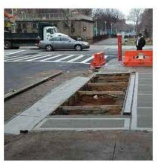
The sidewalk and curb that were removed for the installation are replaced in kind. The new curb has one or two curb cuts that allow water to flow in and out of the bioswale.
