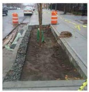
The engineered soil contains sand, which allows for quick infiltration. The soil is graded to allow water to pond at the center of the bioswale during a rainstorm.
