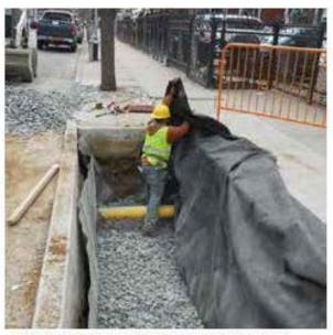
The excavated bioswale is back filed with broken stone, which is wrapped with geotextile fabric to prevent the next layer of soil from dogging void spaces in the stone layer.
