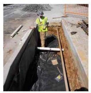
If private utility service lines run through the bioswale, they are fitted with a protective sleeve.
