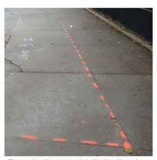
The contractor spray paints the length and width of the bioswale on the sidewalk. These borders are then cut with a saw.
