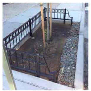
A steel tree guard is installed to protect the plants from foot traffic on the sidewalk. The tree guard posts are set in a concrete footing for stability.
