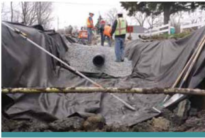
Figure 9.2.9: At the Lakeview Project a gas line was found to span the bioswale trench. Moving the gas line was not an option. An adaptive approach using avoidance was determined to be the best course of action.
