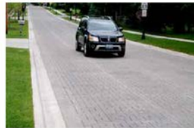
Figure 2.4.5: Permeable pavers can be used in a curb-to-curb application, as shown in this example from Warrenville, IL. Using pavers within the road or along the parking lanes helps with traffic calming. (Source: ICPI)
