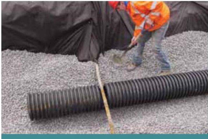
Figure 9.2.10: The above photo shows how the perforated pipe was installed around the exposed gas line at the Lakeview Project. A notch was cut in the perforated pipe and fit into place below the gas line. (Source: Aquafor Beech)
