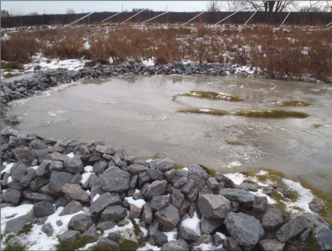
Rip rap check dam to reduce velocity of surface runoff
