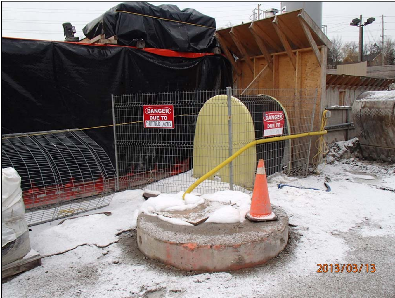
Acid dosing at Shaft 1 muck pond enviro tank
