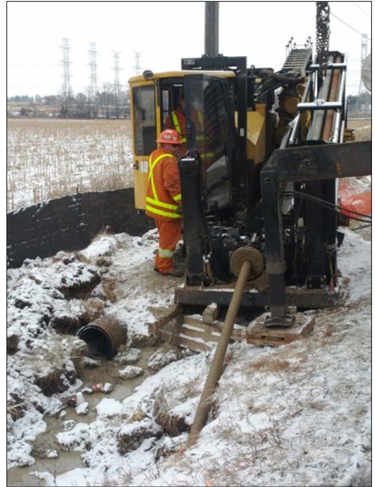
Horizontal Directional Drill rig installing SEP watermain pipe along Altona Rd
