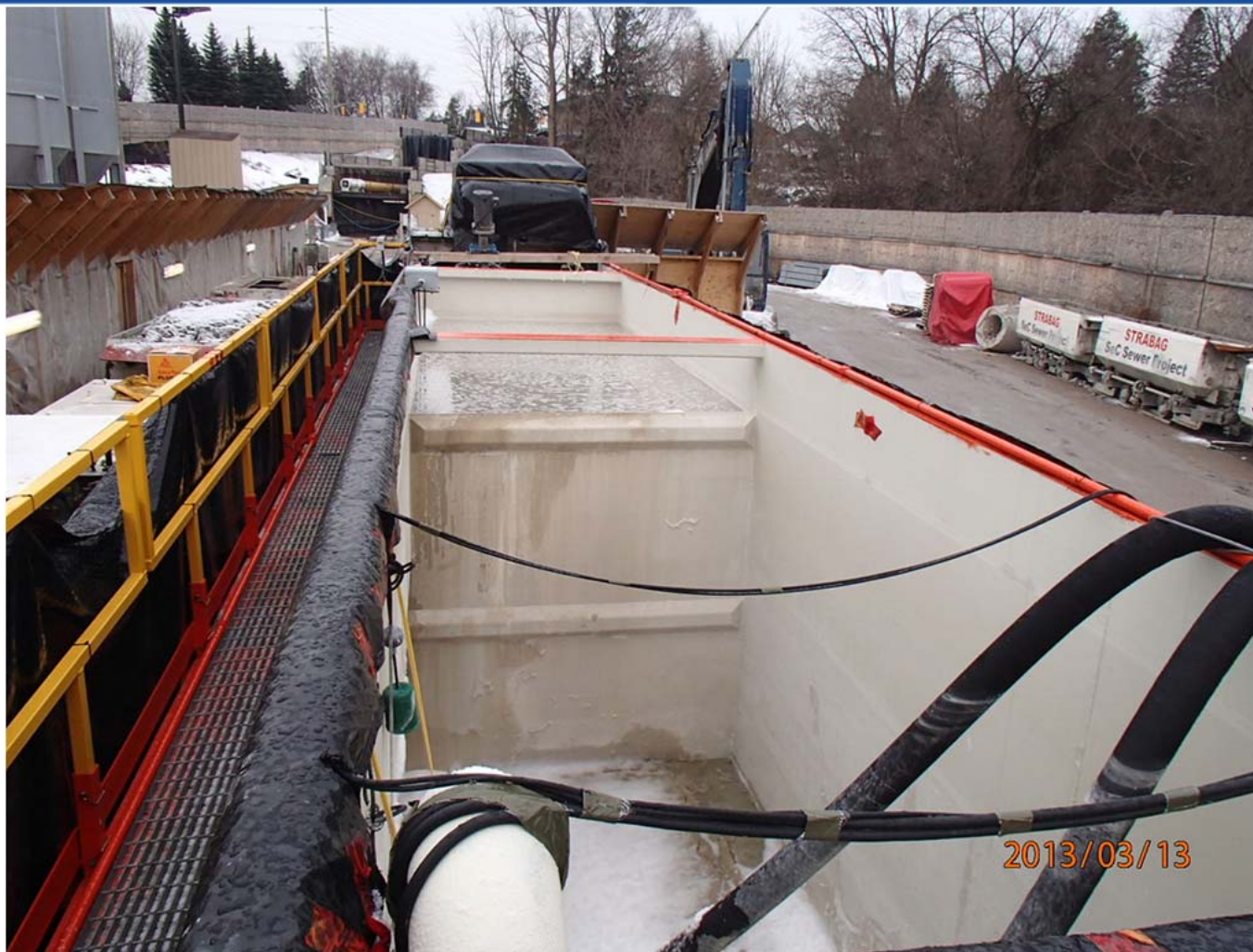
Water control baffles inside SEP envirotank
