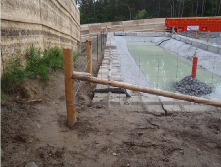
Muck pond with enviro-tank system at Shaft 4
