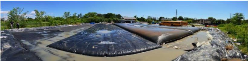
Sediment Removal: The Geotube<sup>®</sup> units were cut open and the consolidated sediment removed and hauled to a disposal site. The sediment is approximately 80% solids in these photos.
