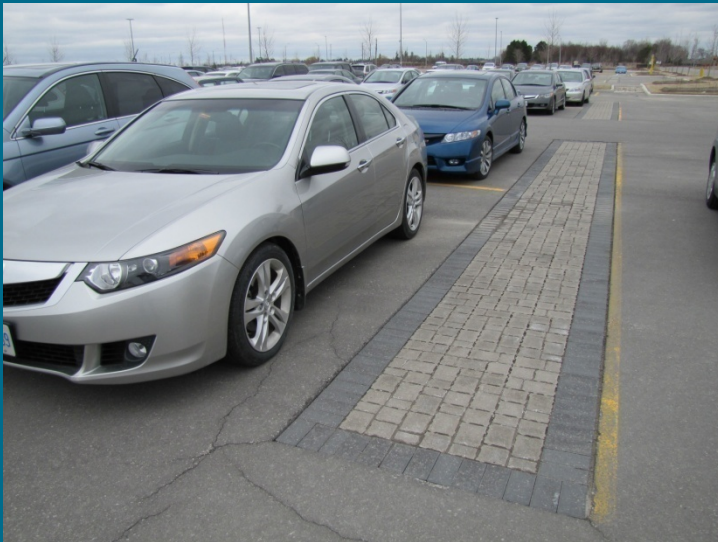
Permeable Pavement in Parking Lot
