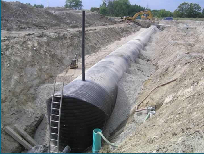
Rainwater Harvesting Tank
