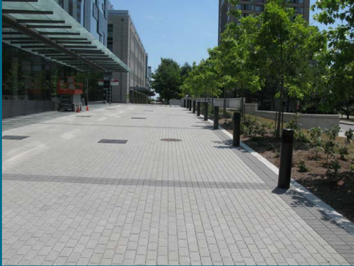
Permeable pavements over rainwater harvesting tank
