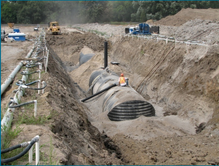
Storage Pipe Construction
