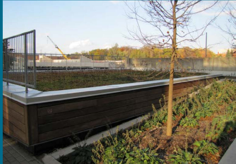
Green roof over top of service area
