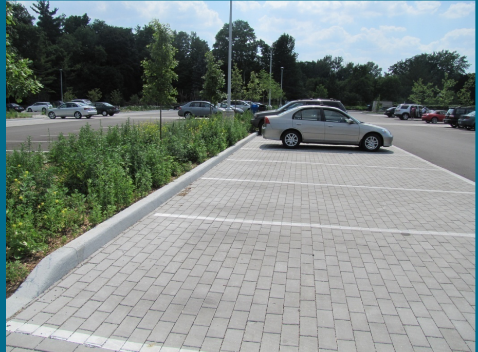
Permeable pavement and biofilter
