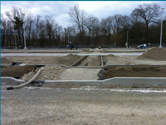
Biofilter inlet and permeable paver installation
