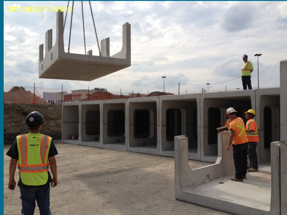
Storage tank installation
