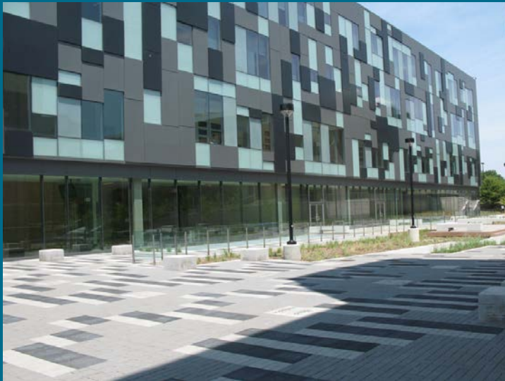
Permeable pavements over plaza over infiltration medium
