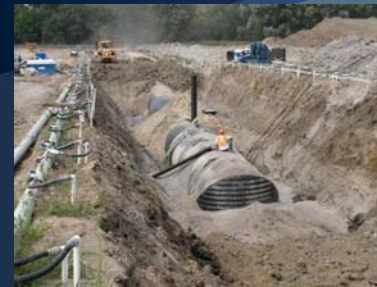
Storage Pipe Construction
