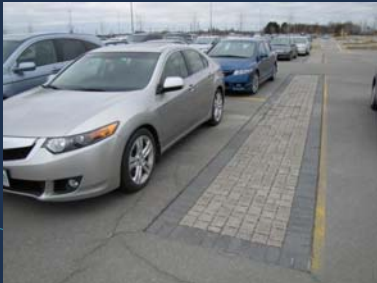
Permeable Pavement in Parking Lot
