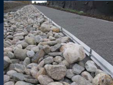
Granular Fitness Path and Drainage Swale
