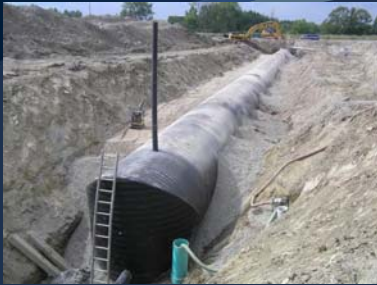
Rainwater Harvesting Tank
