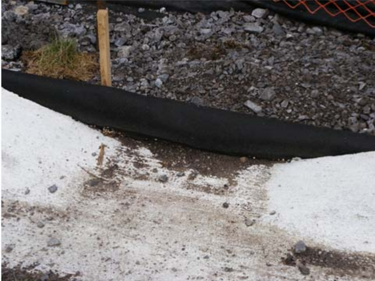
Inlet ESC Controls
