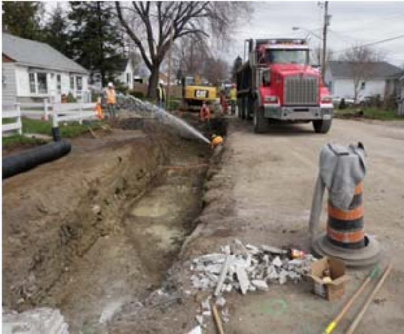
Water Service Line Punctured
