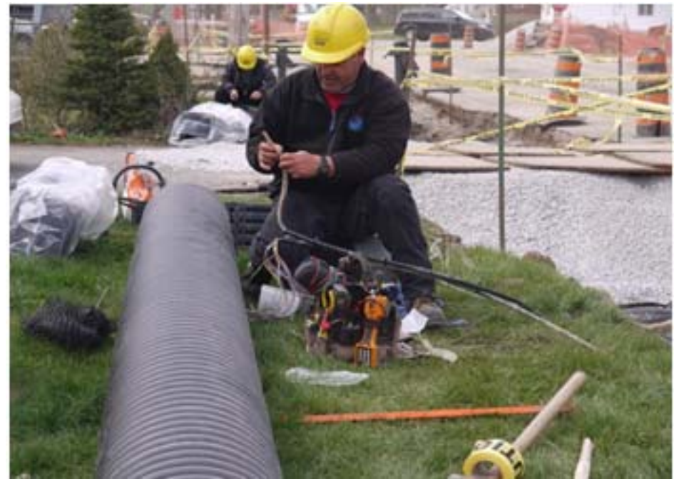
Bell Line Damaged (Bell Service Onsite)
