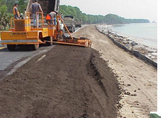
Polymer Enhanced Soft Armor Systems was chosen. After grading, compost was placed as an organic layer
