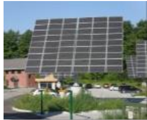
58 kW solar trackers
