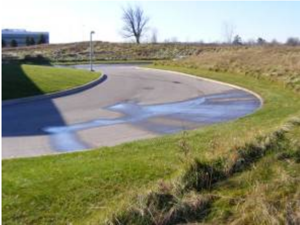
Correcting drainage Issues
