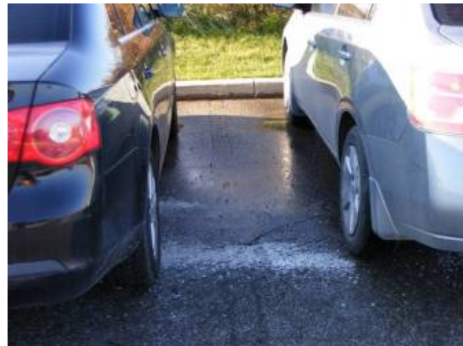
Need for excessive salt application
