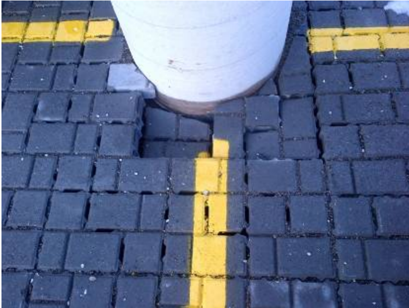
Compaction around light standards
