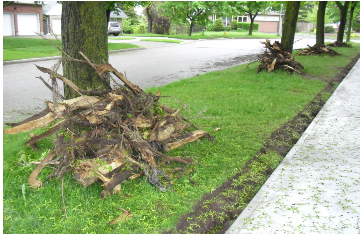
Sidewalk replacement due to damage from tree roots
