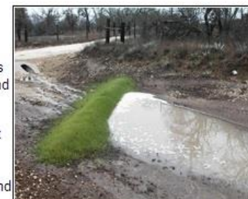
Vegetated compost filter berm. Note sediment on upstream side of berm and clear water on downstream side. Source: S. McCoy, Texas Commission on Environmental Quality.
