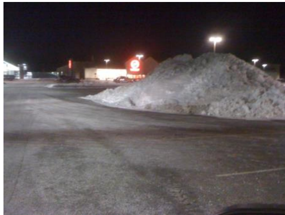
Porous asphalt modest salt and very little black ice , Jan 23, 2011; *note use of PA as snow dump because of positive drainage
