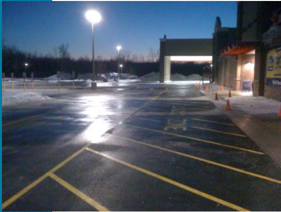
Standard Asphalt HEAVY salt usage and black ice formation, Jan 23, 2011
