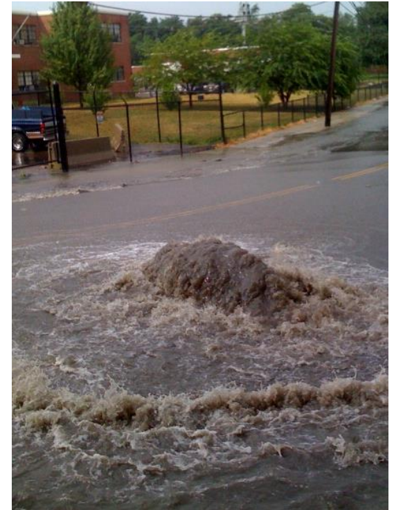
Sanitary/Storm Sewer Backup
