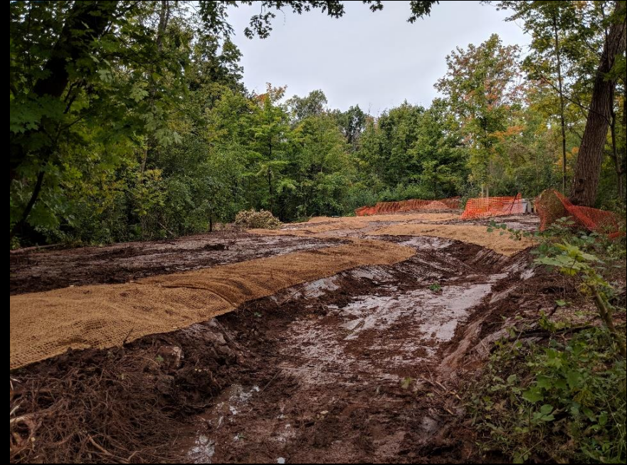
Adjustment of channel geometry to preserve trees
