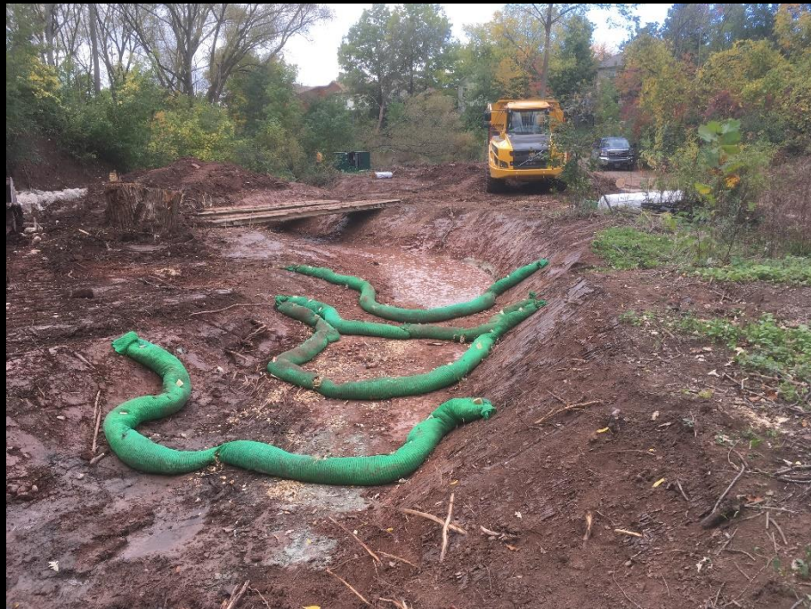
Phase 3: Flow filtered through silt socks
