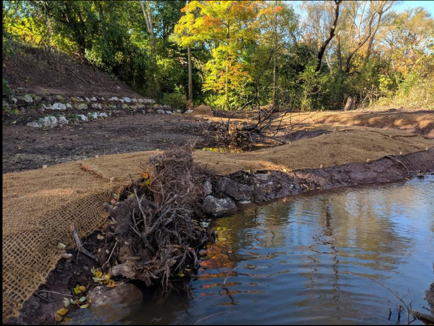
Flexibility in sizing of habitat features to make use of materials harvested on-site
