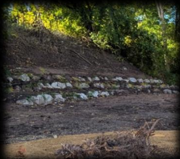
buried vegetated stone buttress
