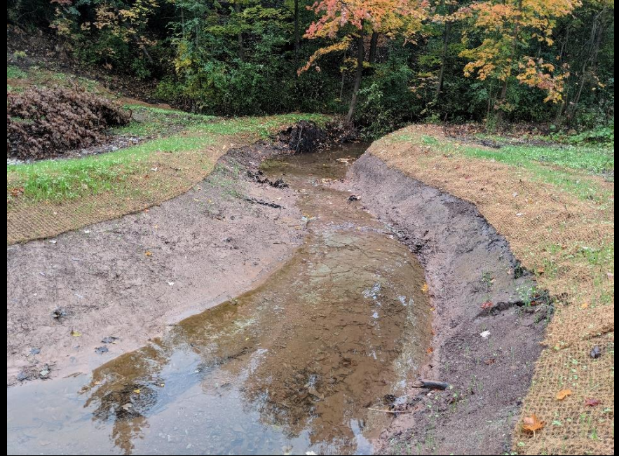
Shale riffle construction
