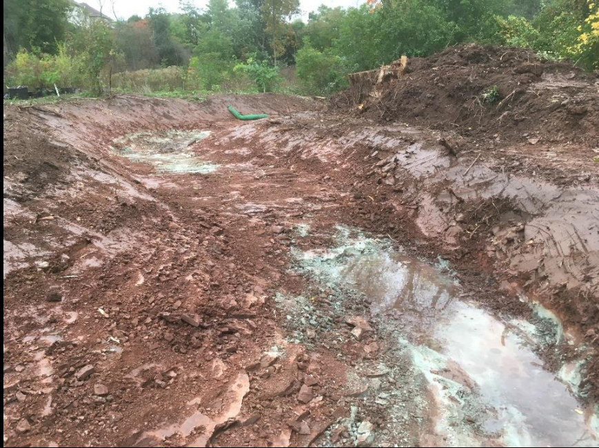
Variability in shale elevation
