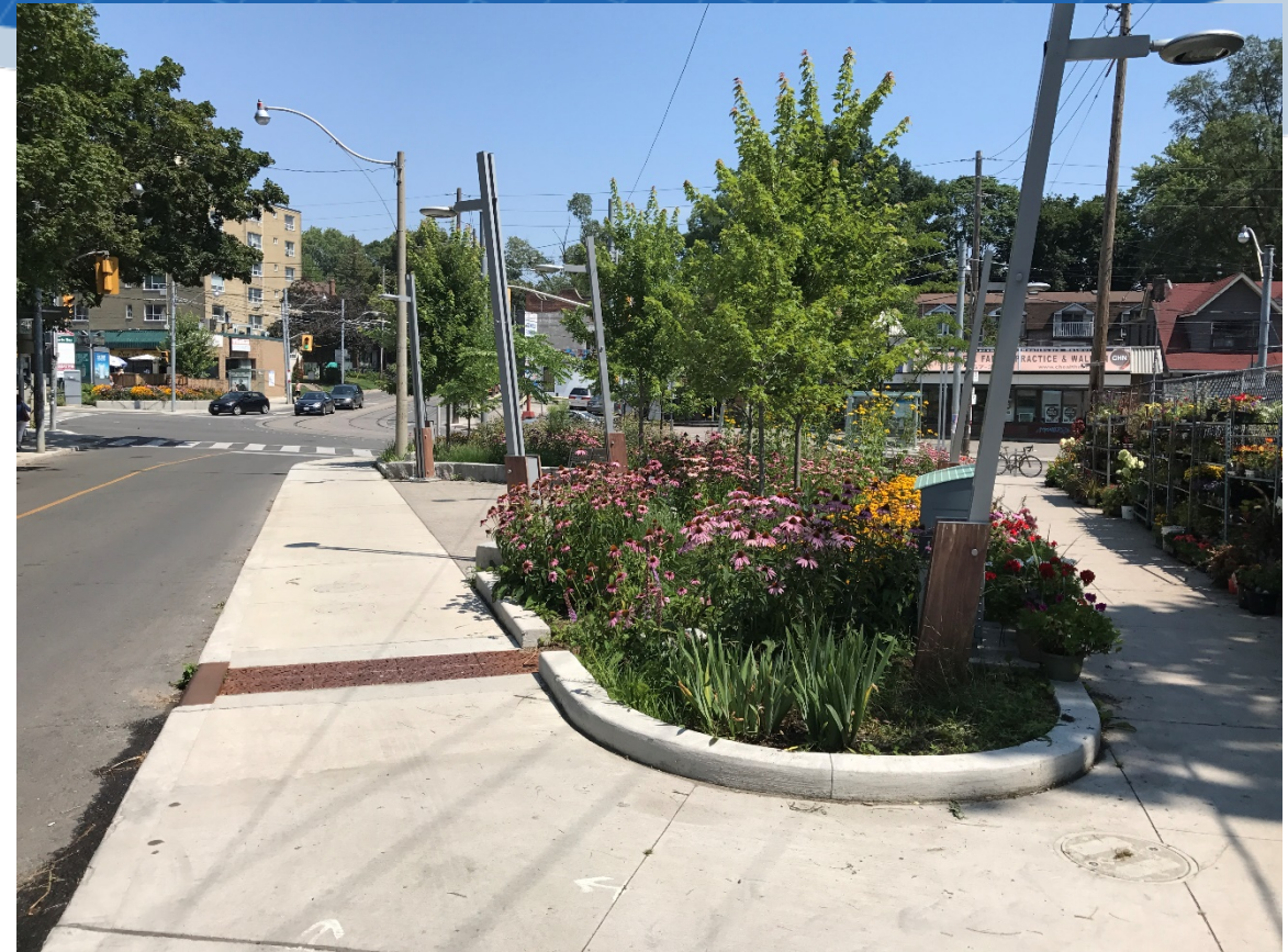
FAIRFORD & COXWELL AVENUE BIORETENTION
