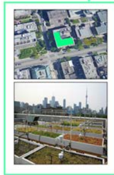
UofT Gritlab Rooftop Modular
