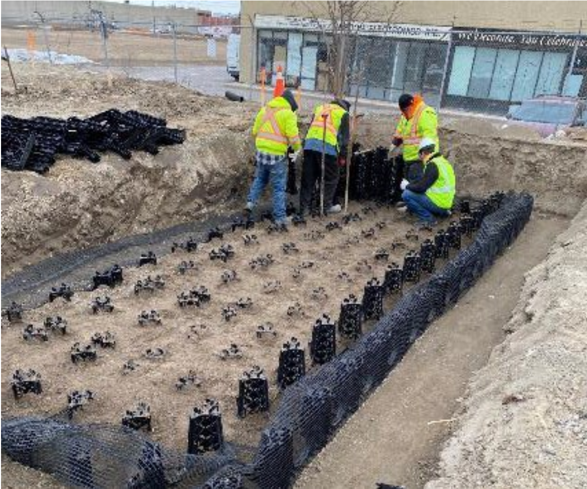
Installation of a Rootspace Plot, Soil Cell Evaluation
