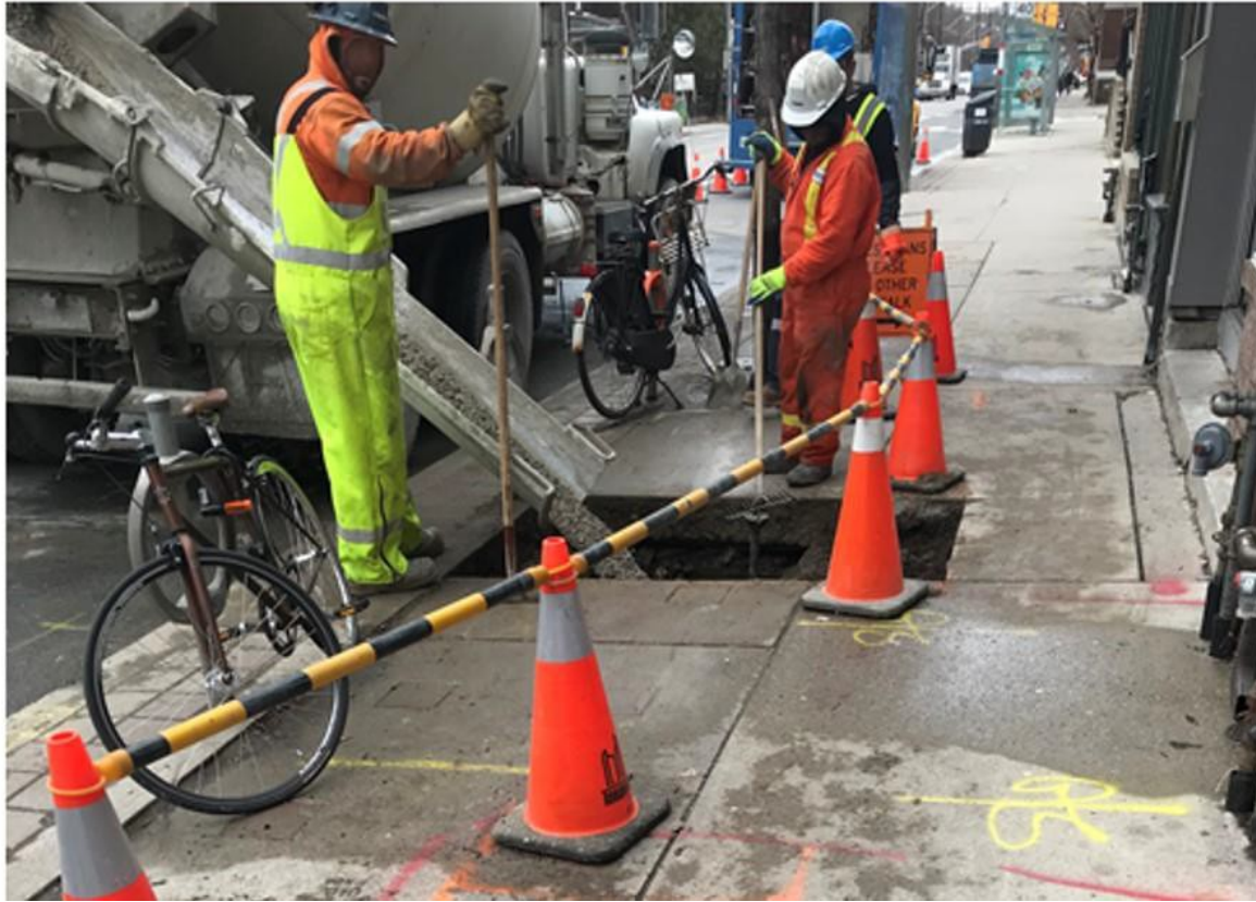
Utility repair, backfilling with unshrinkable fill
