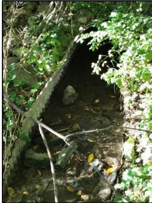
Pipes and Culverts
