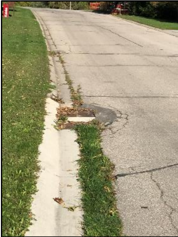
Curbs and Gutters
