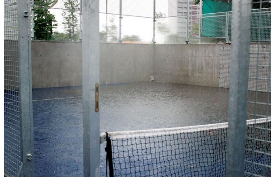
The WATER PLUS project in Gladsaxe is normally used as a paddle court but with heavy rains can also detain and store water © Christina Geer Sørensen
