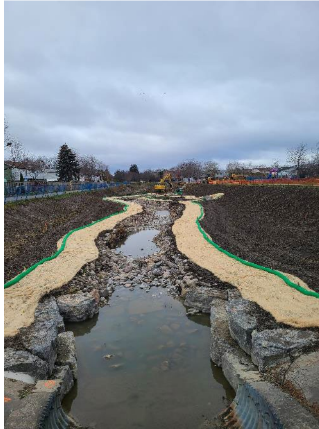
New channel immediately post-construction
