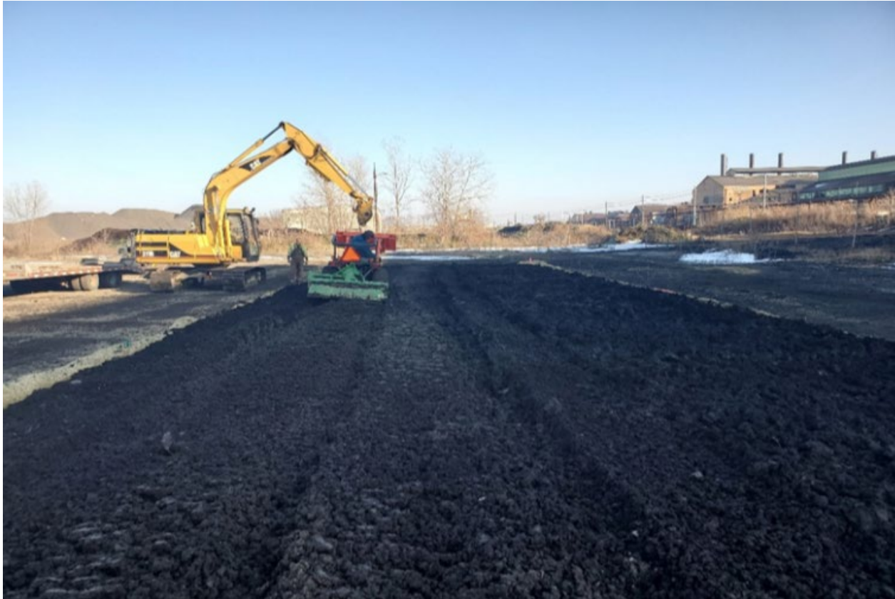
Engineered Fill Evaluation – Cement Stabilized – 3%, 7%, 10%
