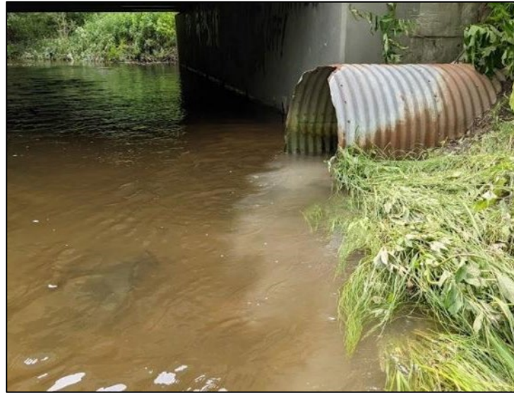
Curb drain (left) and end of pipe (right) showing sediment rich stormwater entering the Wye River during a rain event at site SWM04 (Heritage Park)
