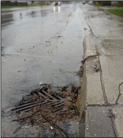
Curb drain (left) and end of pipe (right) showing sediment rich stormwater entering the Wye River during a rain event at site SWM04 (Heritage Park)
