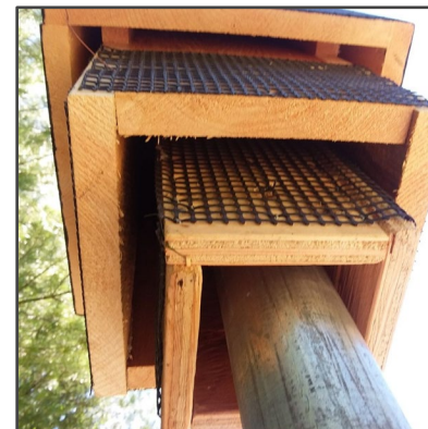
Separate Chambers within Typical Bat Rocket Box
