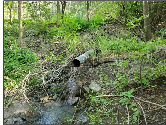
Hanging Pond Outlet Culvert
