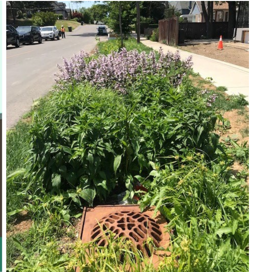
Green Infrastructure: Bioswale Location: Byng Avenue, Etobicoke
