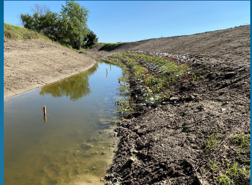
Vegetated Rock Revetment – After Construction
