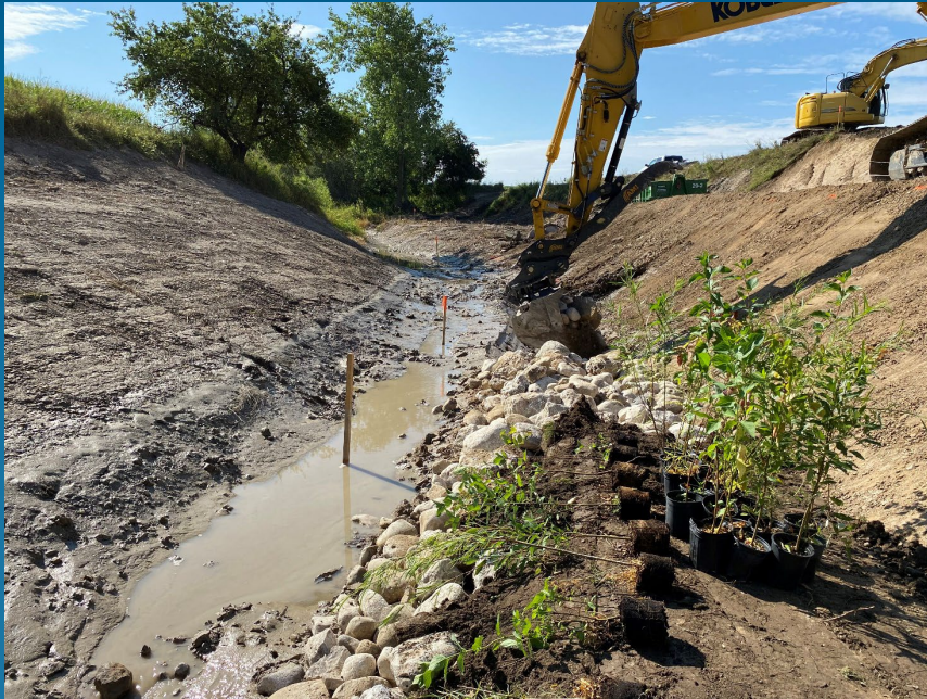
Vegetated Rock Revetment – During Construction
