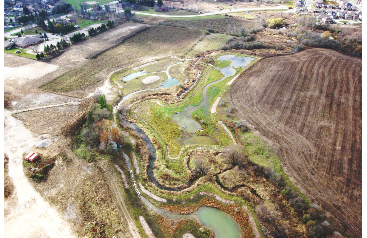
Stoney Creek Flood Control Facility London, ON
