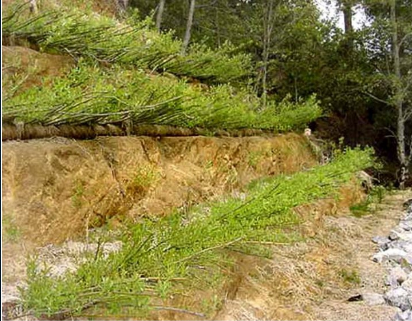
Brush layering along a steep slope. (California Department of Transportation: http://www.dot.ca.gov/ )
