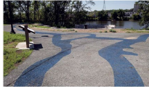
Edgewater Park in Minneapolis is designed to be sustainable, with prairie grass and native plants chosen for their low maintenance and their ability to capture storm-water. The pervious concrete fits right in. It's stained blue in places to mimic the paths of the nearby Mississippi and Minnesota rivers. Photo courtesy of Cemstone.
