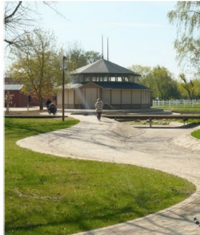
Small hills in the tile paving - inlets for regular rainfall
