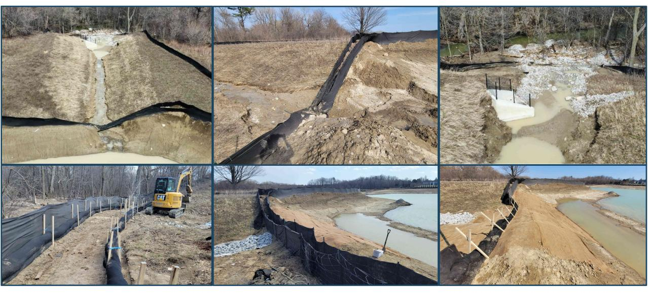
⊗ Clogged geotextile at ESC Pond EOW retained excessive run-off - resulting in catastrophic silt fence collapse.
