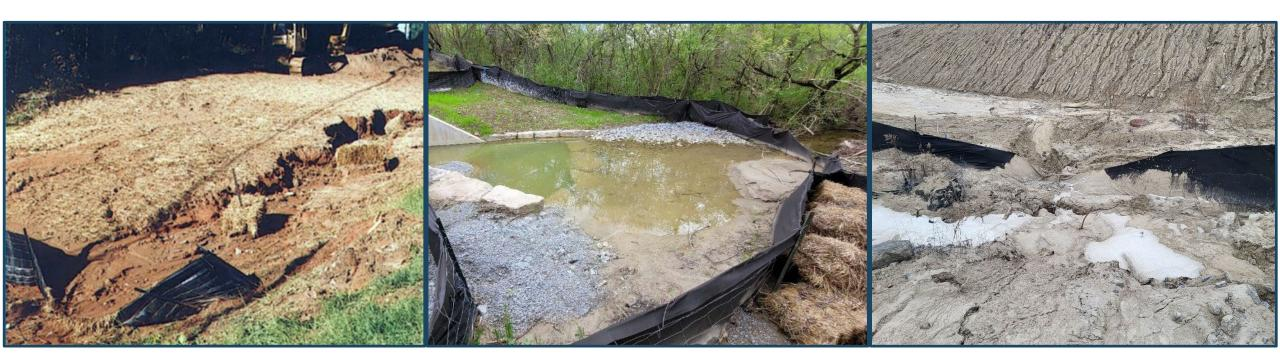
Oouble row wire-backed silt fence with straw bale support is more costly than double row 300 mm filter sock with page wire fence. Even before repairs / restoration. Must be replaced when clogged (rarely done);
