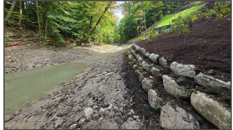
Vegetated Buttress and Channel Substrate Integrated into Armourstone Retaining Wall
