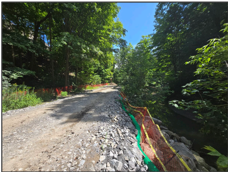
Heavy Duty Access Route During Construction
