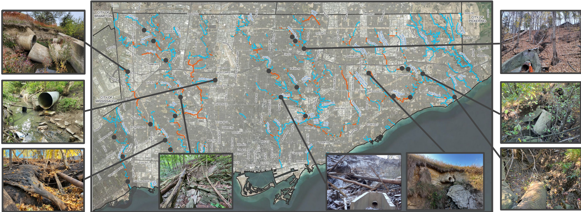
Numerous Drastically Failed Stormwater Outfalls Across Toronto
