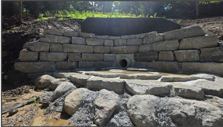
Grouted Armourstone Scour Pad
