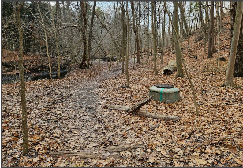
Sanitary Sewer Network Present Along Access Route
