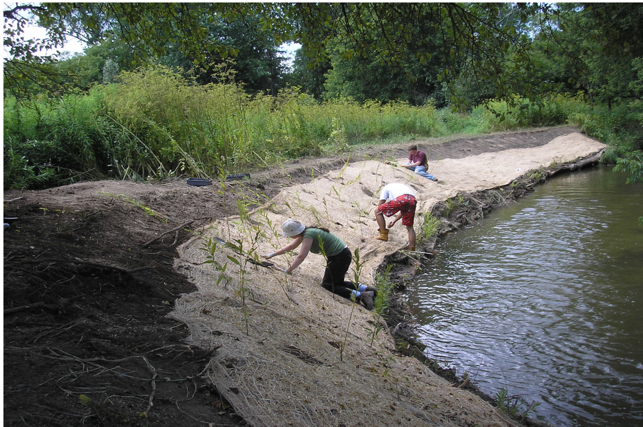
Slope seeded with grass seed, covered with coir and shrubs planted
