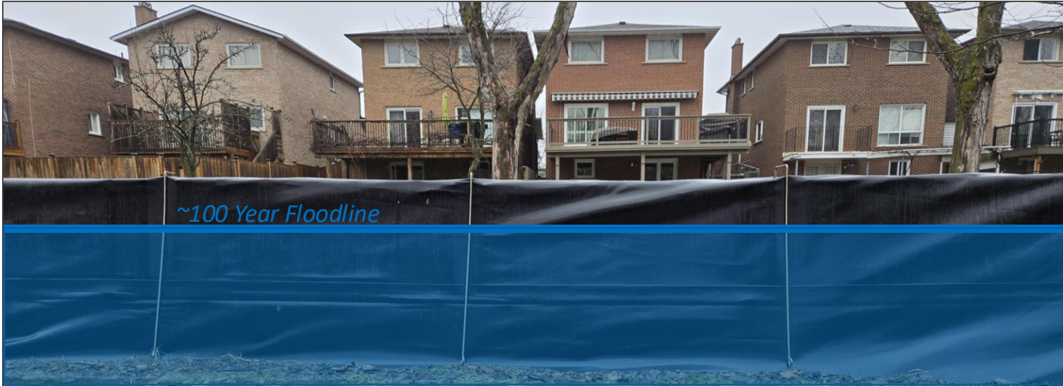
Floodwall Protection Provided to Private Properties
