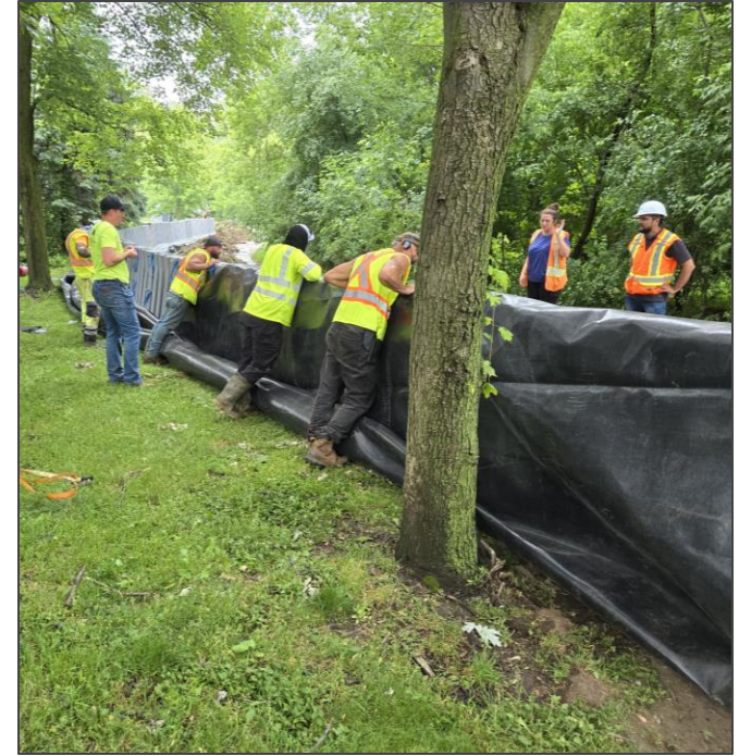
Onsite Floodwall Installation and Maintenance Training
