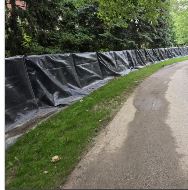
Completed Floodwall After Restoration
