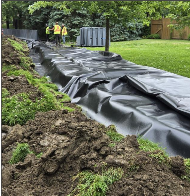
Trenching and Liner Installation
