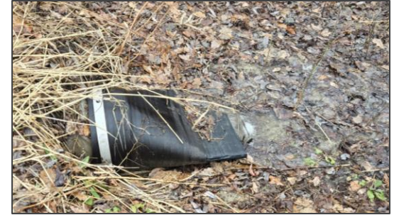
Backflow Preventer Attachment on Culvert
